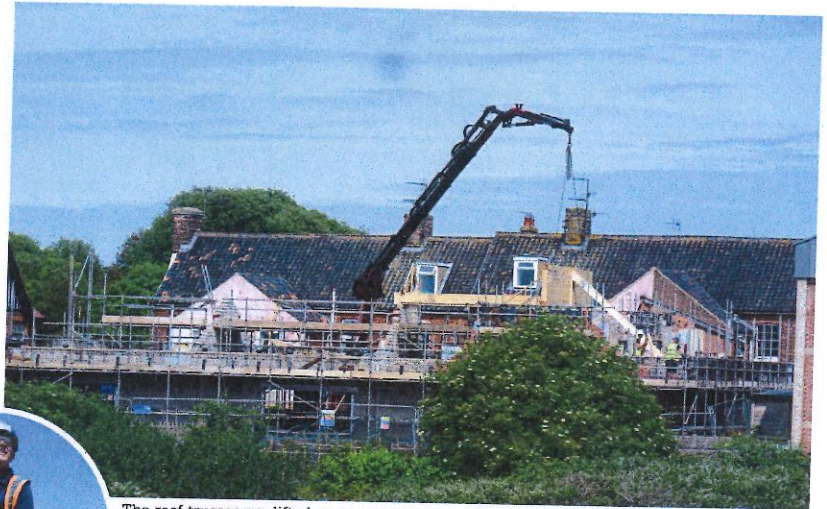
The roof trusses are lifted on as construction of The Hub - a new workspace at Southwold - reaches the halfway point.
